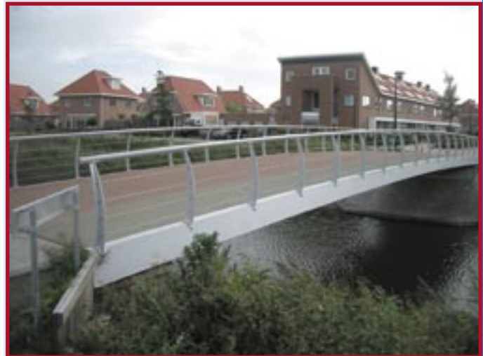
All composite Bicycle Bridge, Dronten. Photo: KCA
