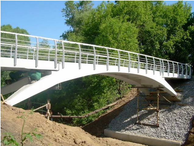
Bridge picture above: Moscow Park "50-years Anniversary of October revolution". Bridge by Apatech, Russia and Light Weight Structures, Netherlands. Length of bridge 22.6 M1, width of bridge 2.5 m1. Installation: July 2008.
