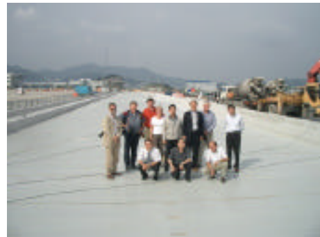
Picture B: Noolcha Bridge
