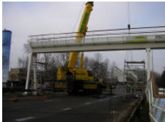
Installing first part and the second part on the background
