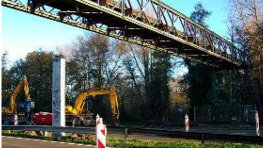
< temporary steel bridge
