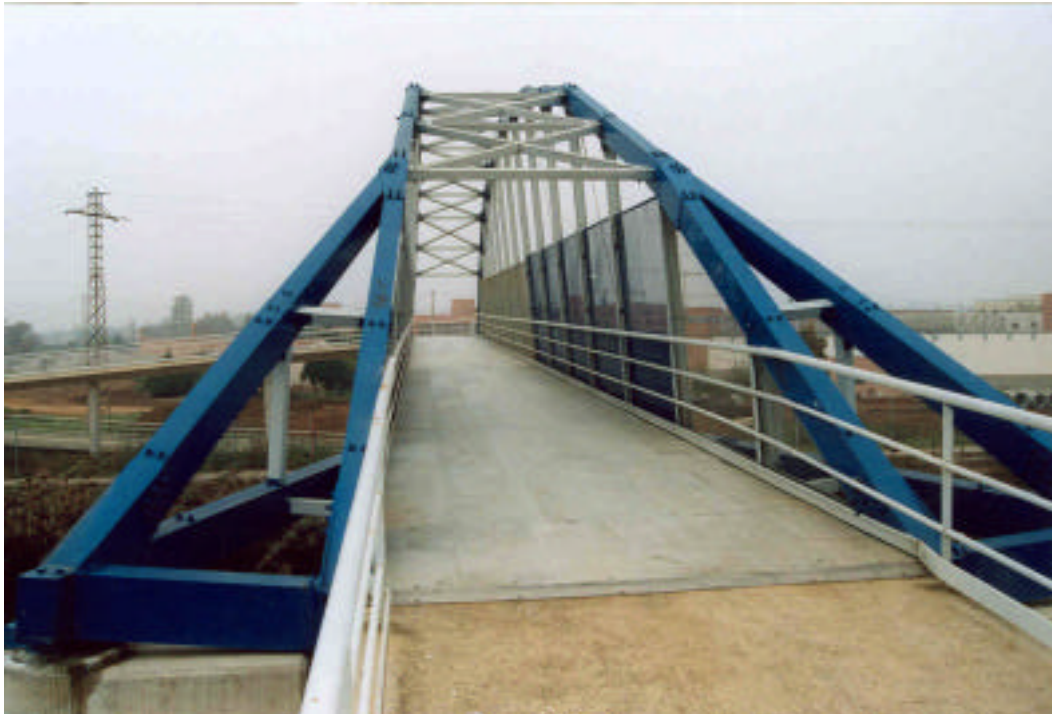
Fig.1. Composite footbridge over a number of railroad tracks in Lerida, span 38 m
