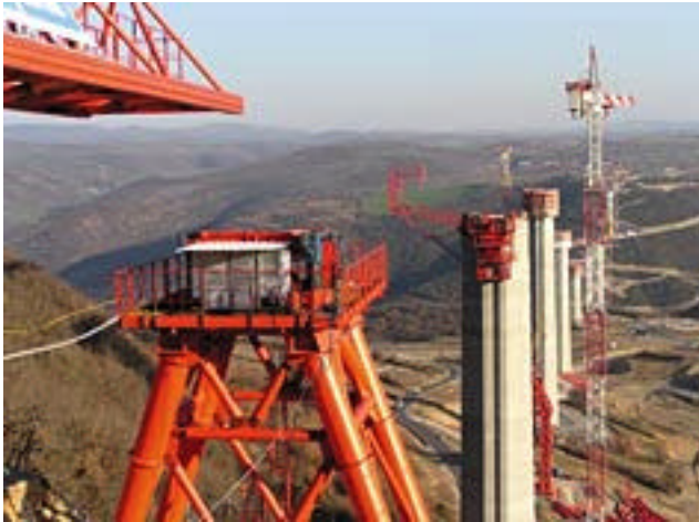
Pier P7 to pier P1.
